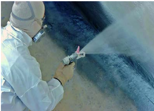
Paint protector of electromagnetic radiation. It is applied to protection against electromagnetic radiation (Germany)
